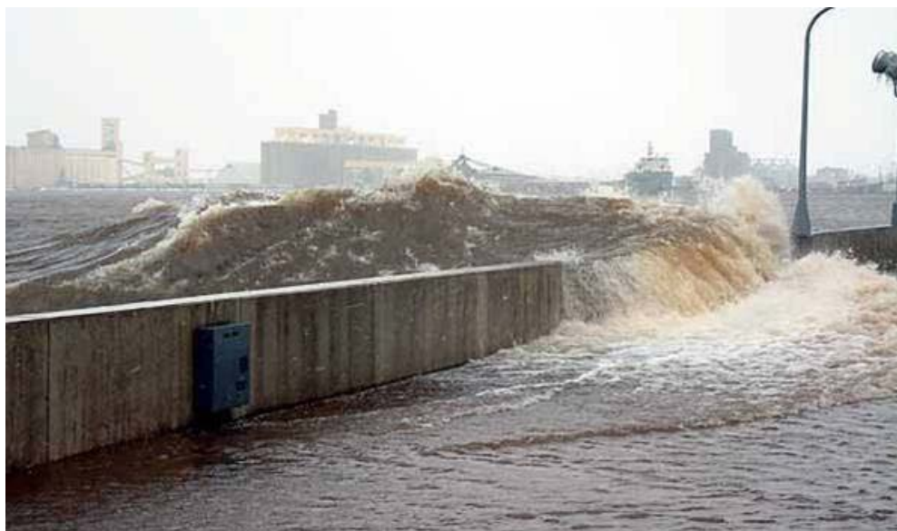
Figure 18. Wind-generated waves overtopping the harbor structure in Canal Park in Duluth, Minnesota. (Gene Clark, Wisconsin Sea Grant)
