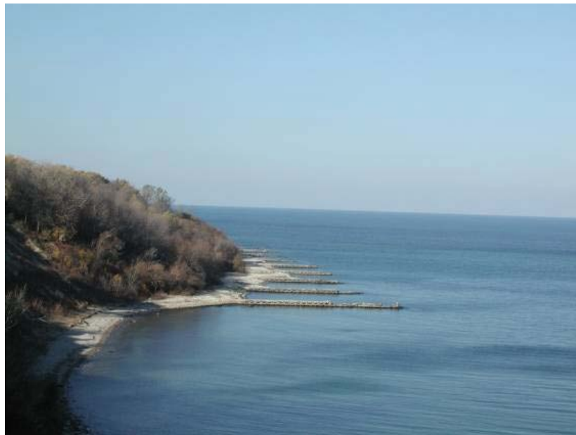
Figure 22. View along the shoreline in southern Milwaukee County showing an old groin field that has been effective at stabilizing the slope behind it (wooded slope). But, partly as a consequence, there has been increased erosion in the area south of the groin field (foreground). (Source D. Mickelson.)
