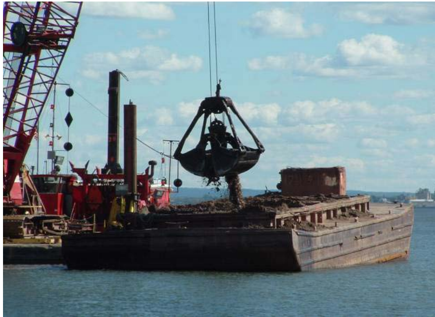
Figure 15. Dredging may be required to deepen channels in marinas during periods of low water. (Gene Clark, Wisconsin Sea Grant)
