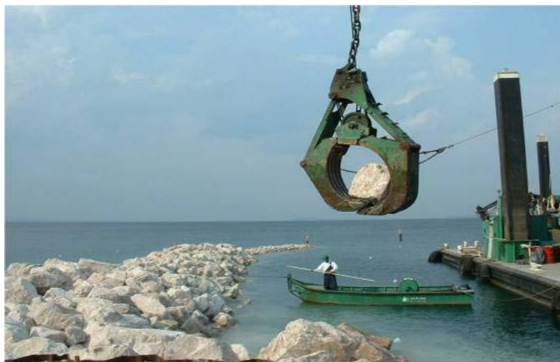
Figure 19. Reinforcing a break wall to better withstand storm surges. (Gene Clark)
