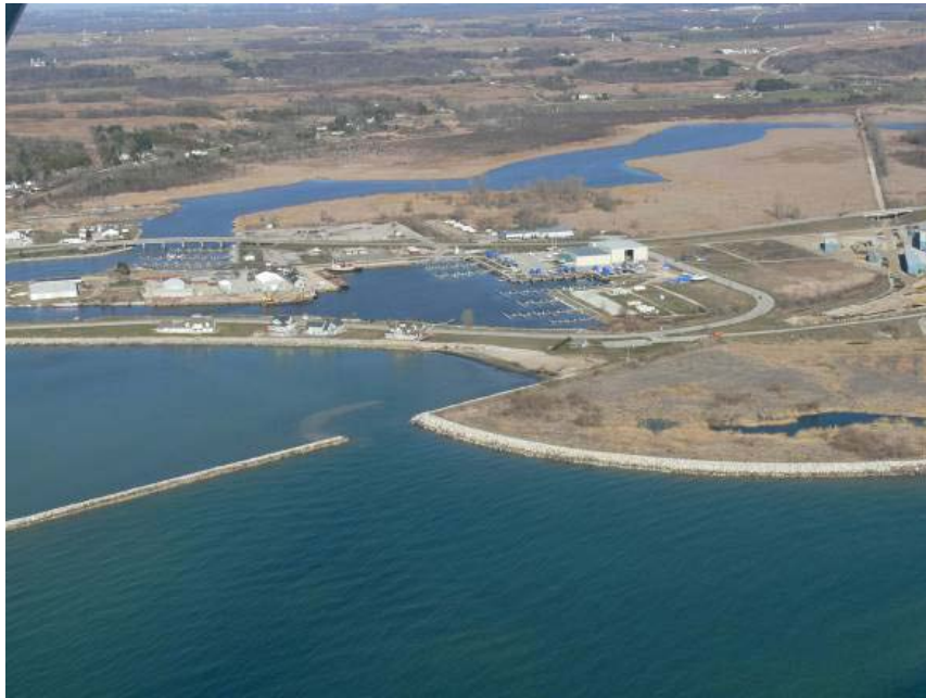
Figure 14. Aerial photo (2007) of the harbor at Kewaunee. This is an example of a harbor that would be affected by substantial changes in lake level (Source: D. Mickelson).
