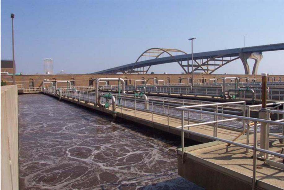
**Figure 4.** Jones Island wastewater treatment plant biological treatment aeration beds. High volumes at the plant following storm events may cause these reactors to washout, which would diminish treatment capabilities. Facility designs may need to consider additional capacity if climate changes alters storm patterns.
