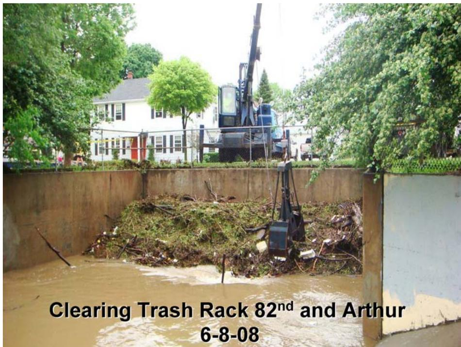
**Figure 3.** Debris from stormwater and flooding in Honey Creek inlet following torrential rains in June 2008. (Photo provided by the Milwaukee Metropolitan Sewerage District)
