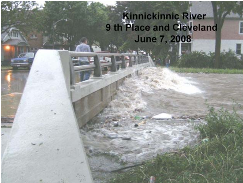
Floodwaters impact Milwaukee neighborhoods following heavy rainfalls, June 7, 2008. (Photo courtesy of the Milwaukee Metropolitan Sewerage District.)
